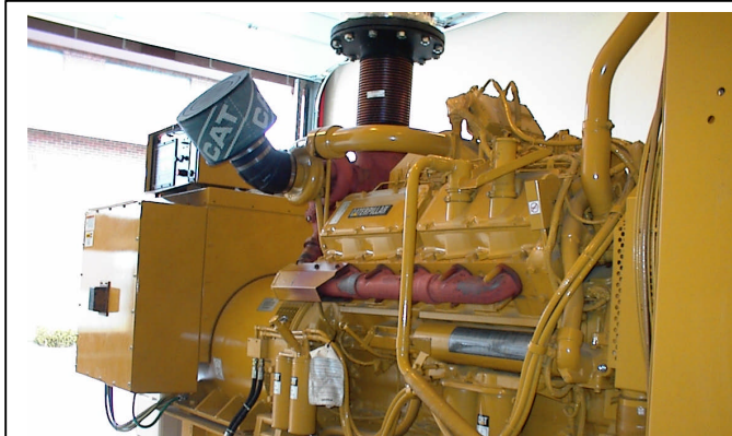
1000 horsepower diesel generator will keep the Water Plant in production during any length power outage. This generator was added to the plant during the chemical building construction in 1999.
