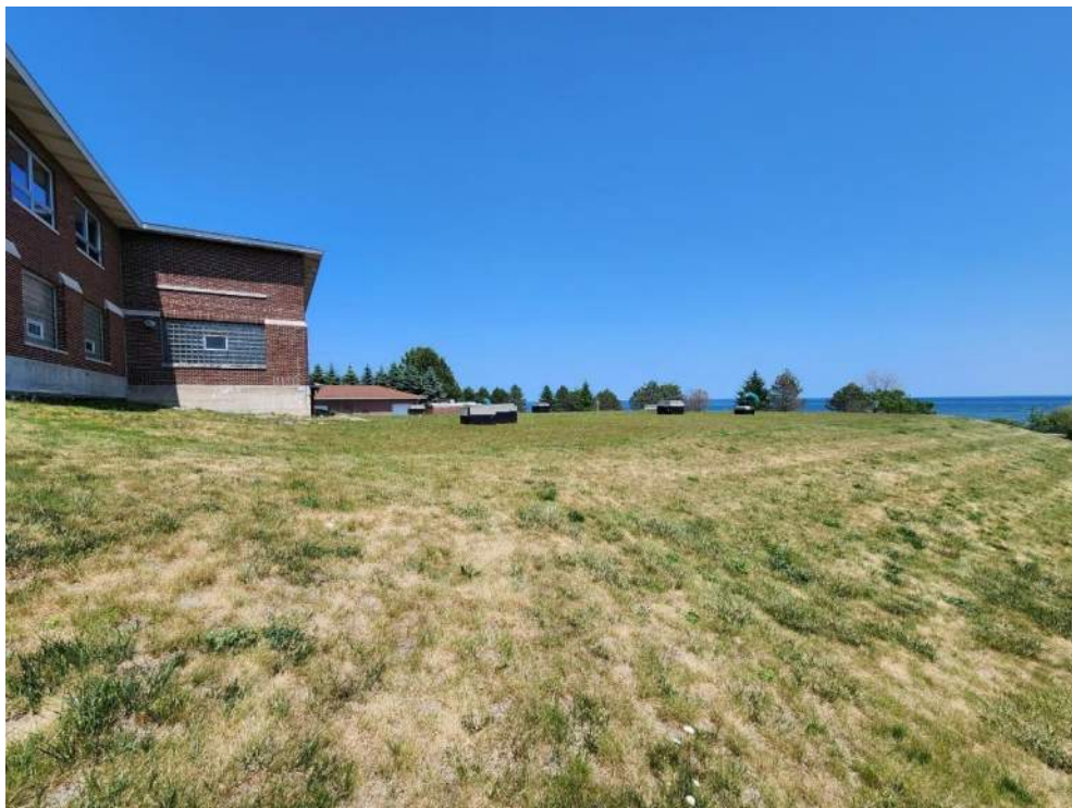
Photograph #1: View of the existing clearwater tank. The view is to the northeast. (Project No. 2023.1089 Alpena Water Production Plant, Alpena, Alpena County, Michigan, March, 2023)
