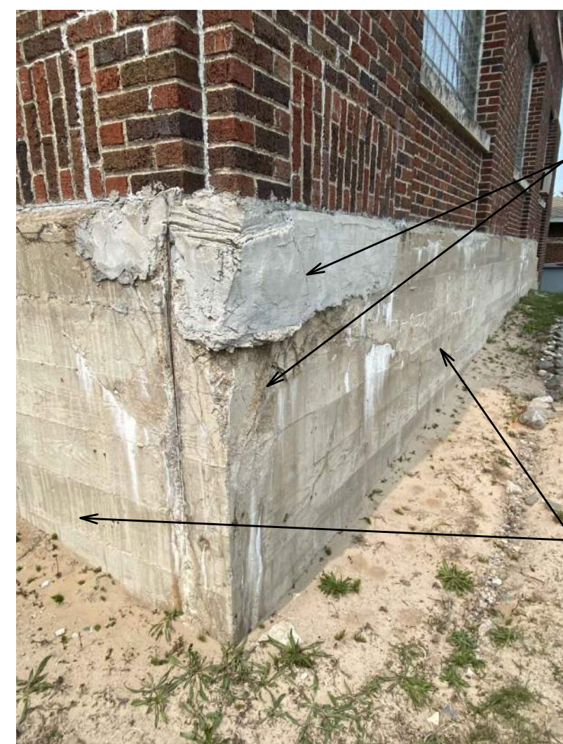
SOUTHEAST CORNER OF ORIGINAL BUILDING
