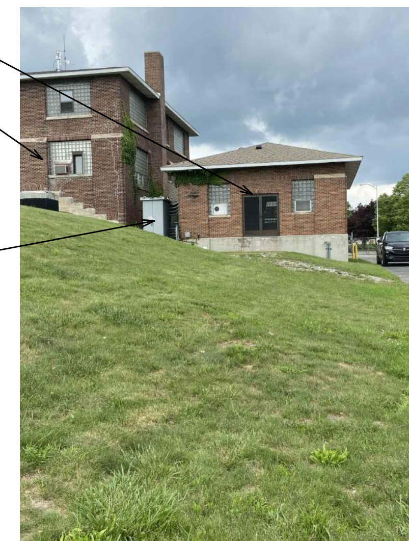
EAST FACE OF HIGH SERVICE PUMP STATION
