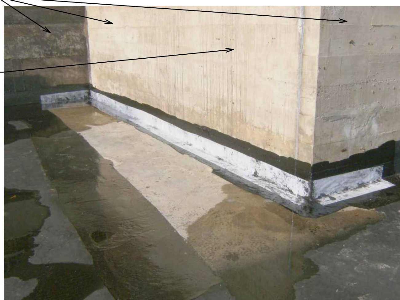
SOUTHEAST CORNER OF LAB WALL FOUNDATION AT TANK
