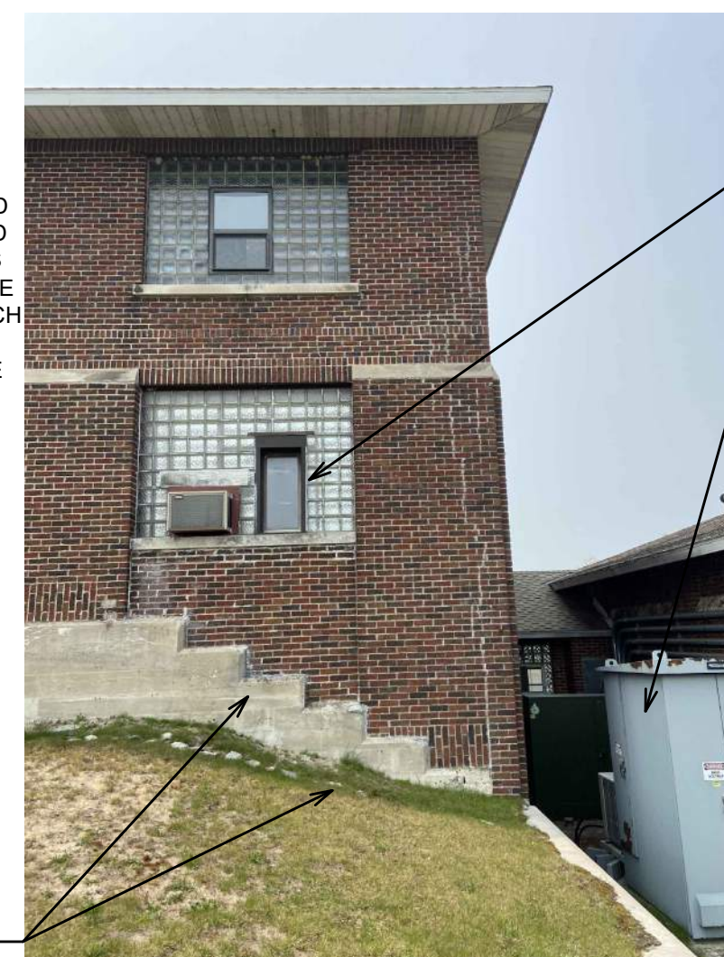
NORTHEAST CORNER OF ORIGINAL BUILDING
