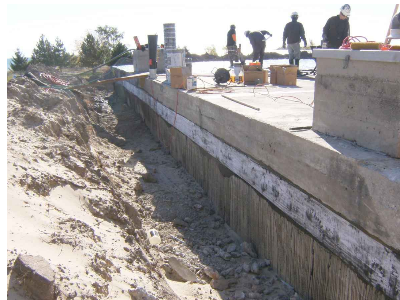
NORTH WALL OF CLEARWELL #1 LOOKING EAST
