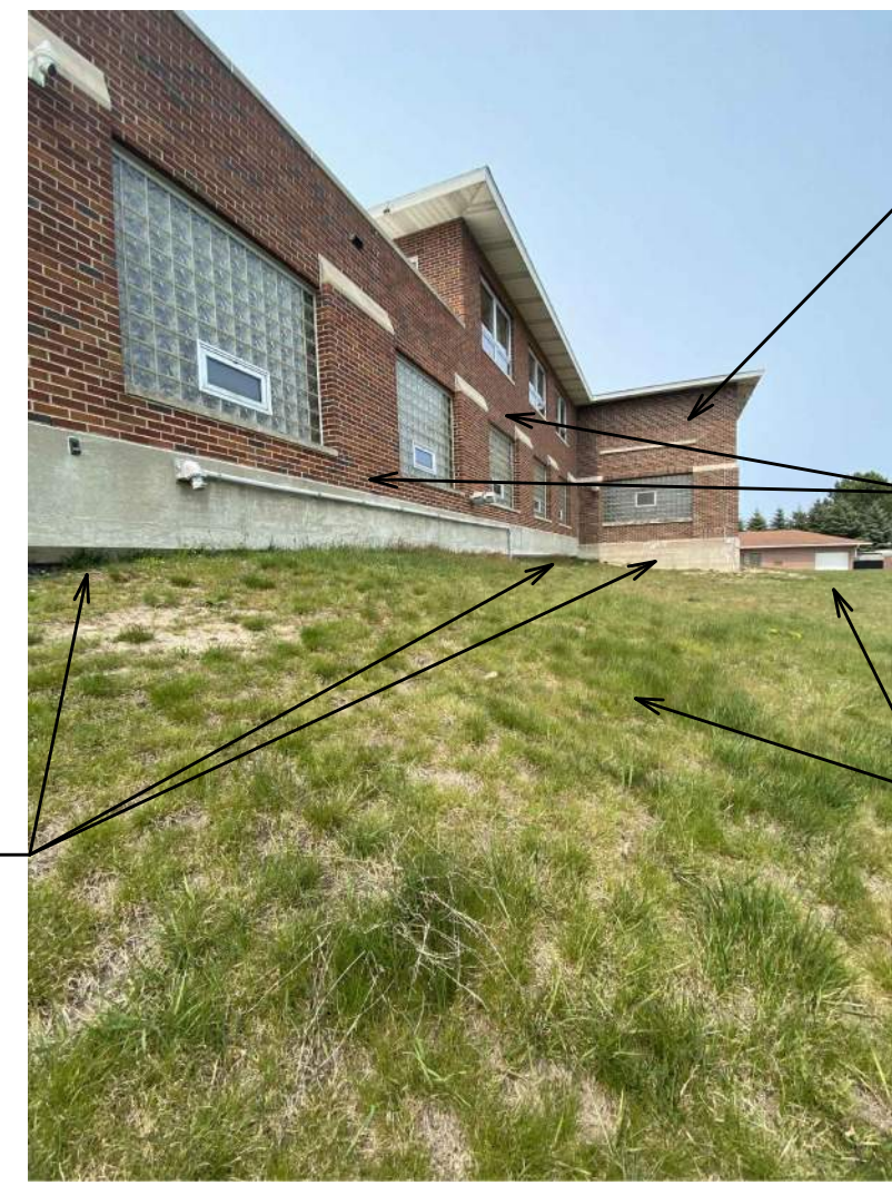
EAST WALL LOOKING NORTH
