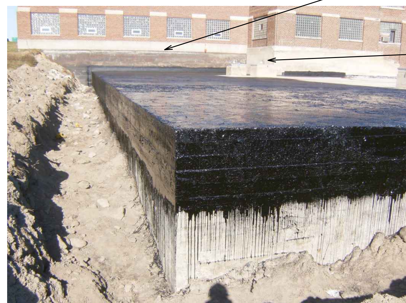
CLEARWELL #2 LOOKING WEST
