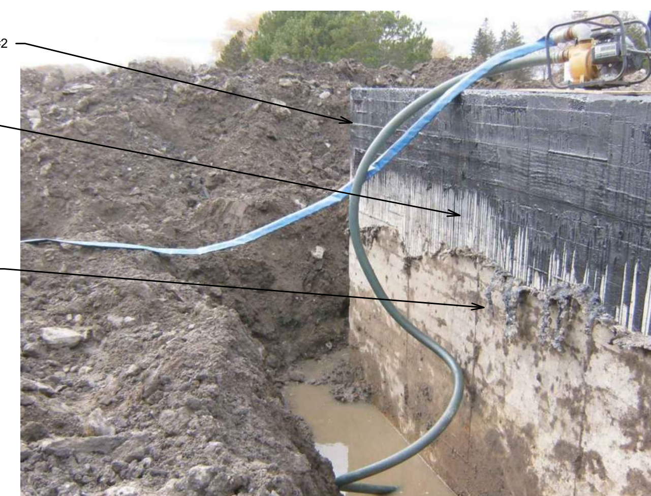
NORTHEAST CORNER OF CLEARWELL #2
