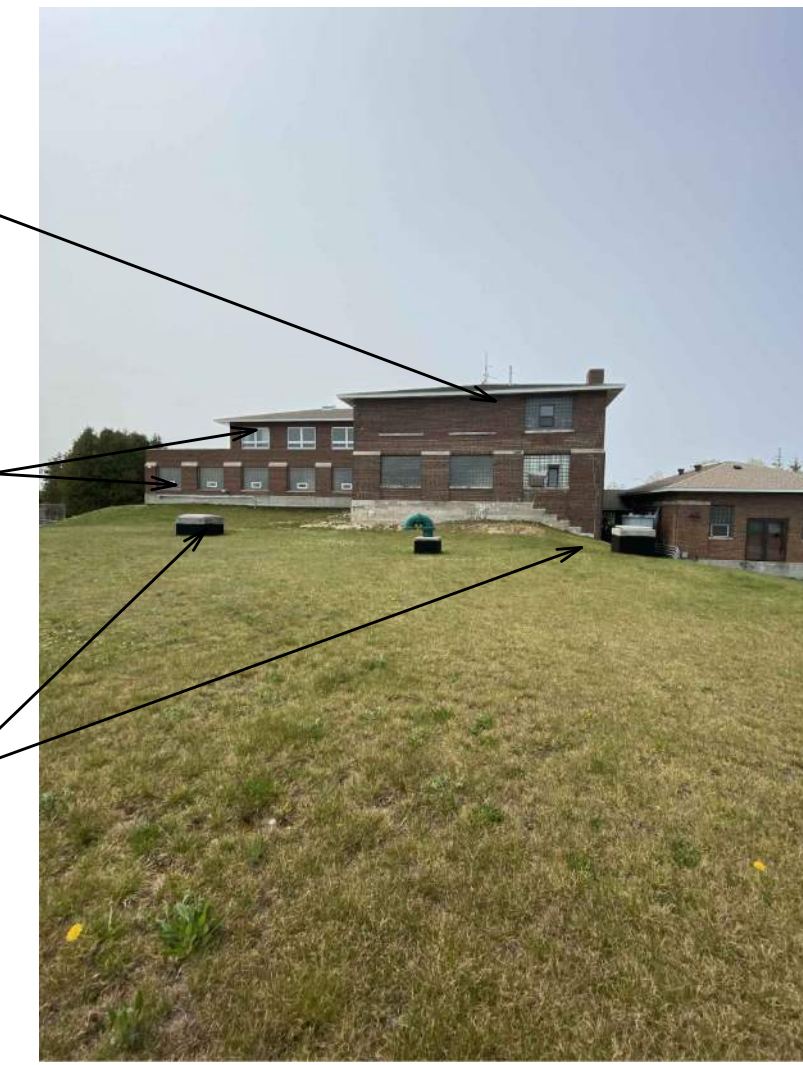
EAST WALL LOOKING WEST
