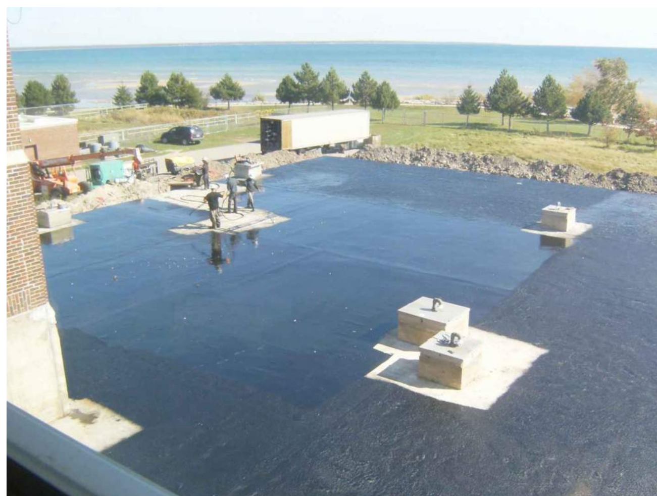
WATERPROOFING UNDERWAY OVER CLEARWELLS
